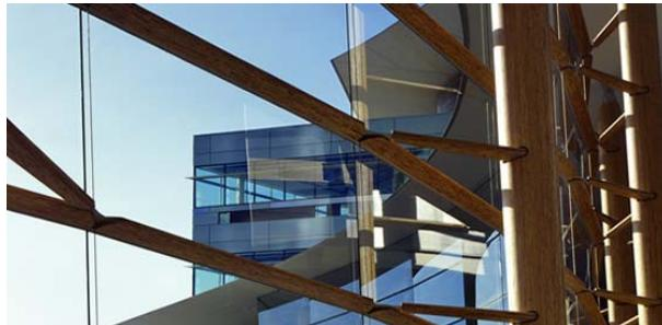
**Figure 11:** Parallel Strand Lumber Columns with support arms and muntins
