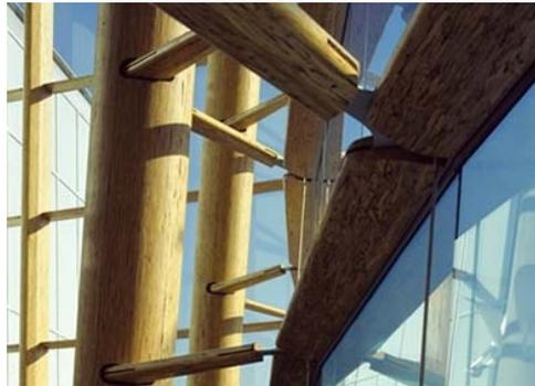
**Figure 16:** Curtain wall similar to Arena Stage (image provided by StructureCraft Inc.)
