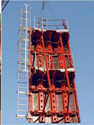
Figure 10: Movement to next lift via crane
