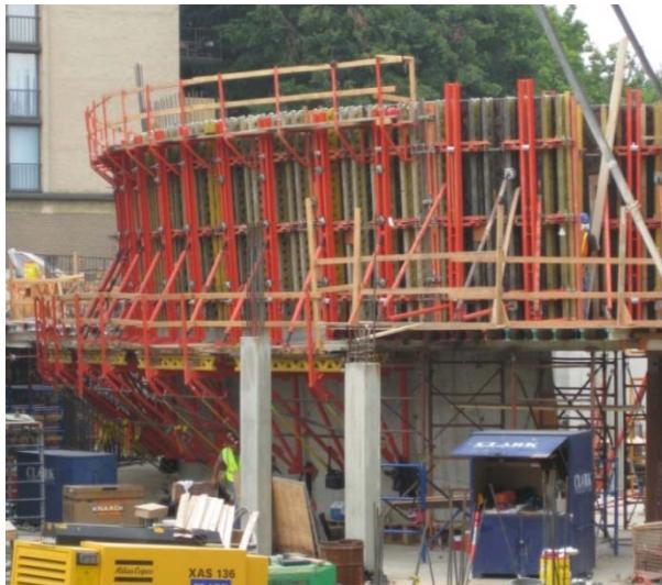
**Figure 9:** PERI RUNDFLEX formwork prepared for a lift pour
