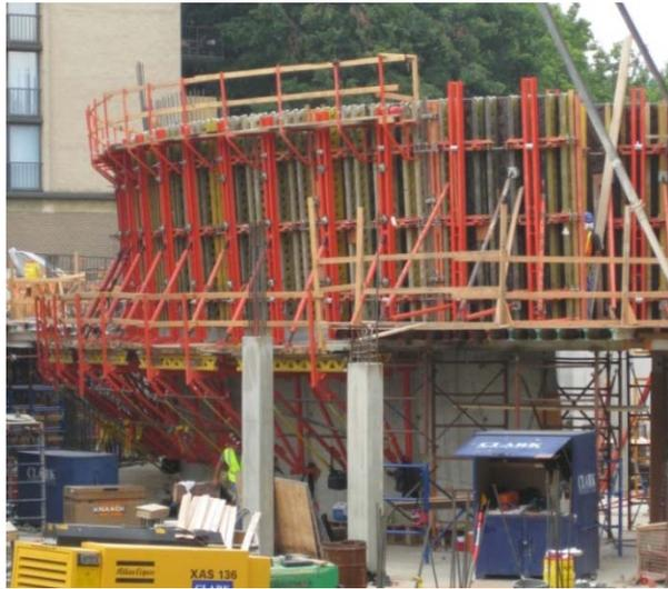
Figure 9: PERI RUNDIFLEX formwork prepared for a lift pour
