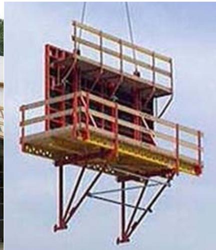
**Figure 7:** PERI CB 240 climbing platform system (Cradle) **Figure 8:** Movement to next lift via crane
