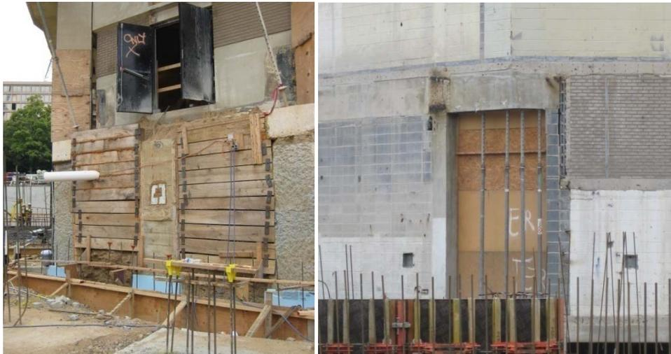
**Figure 14:** Fichandler Underpinning (left) and Kreeger above-ground shoring (right)
