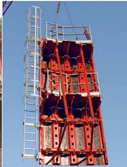
**Figure 10:** Movement to next lift via crane
